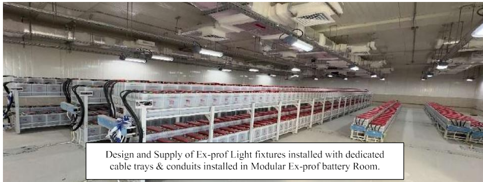
Explosion Proof Battery Room with Explosion Proof Lighting System
