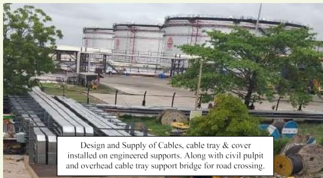
External Cabling System on Cable Trays
