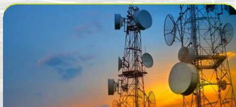
Power and Telecommunication
