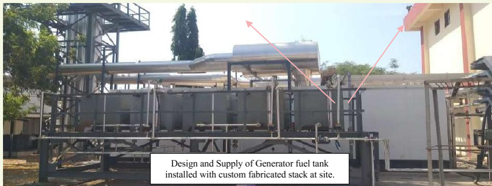
Fuel Tank for Generators
