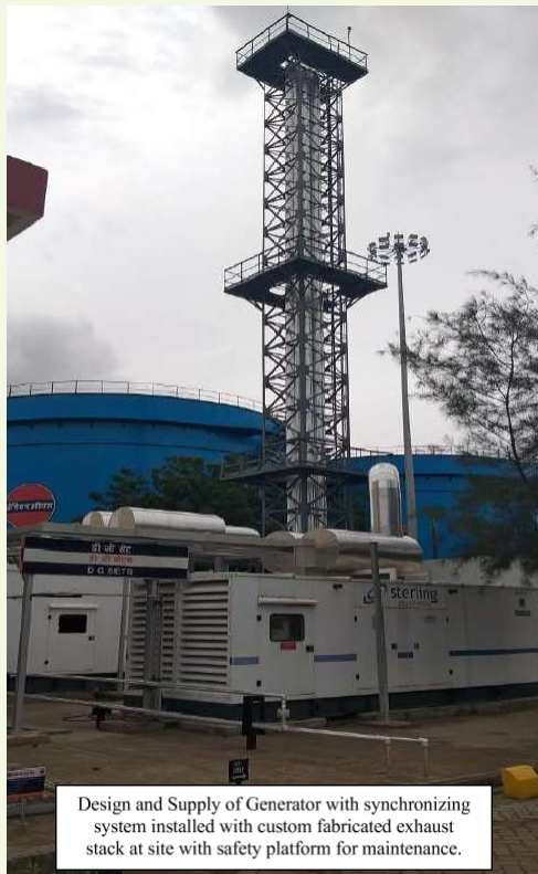
Generator with Exhaust Stack
